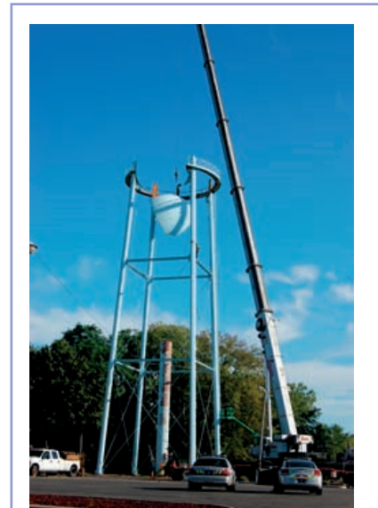
Union’s water tower dating to 1959 was dismantled in July.
