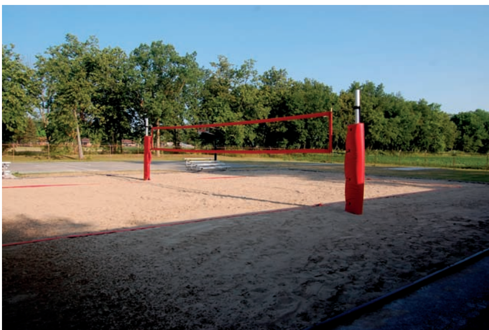
New volleyball court! We've just installed a sand volleyball court at Parkgrove Park (former city pool site). Two cornhole courts are near completion at the facility, and a basketball court was installed last year.
